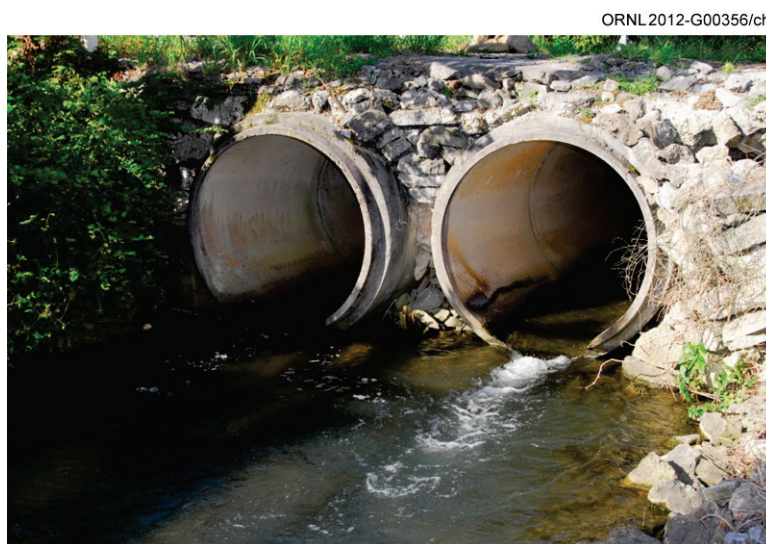
Fig. 4.47. Contaminated storm sewers were the primary source of mercury contamination in Poplar Creek.
