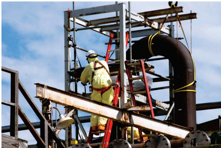
Fig. 4.46. Building 9206 Filter House Removal Operations.
